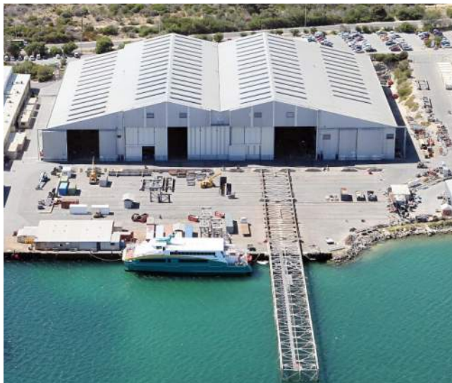
AUSTAL SLIPWAY, HENDERSON
